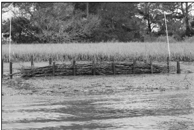
Installation of the gabion-breaks during pilot study
