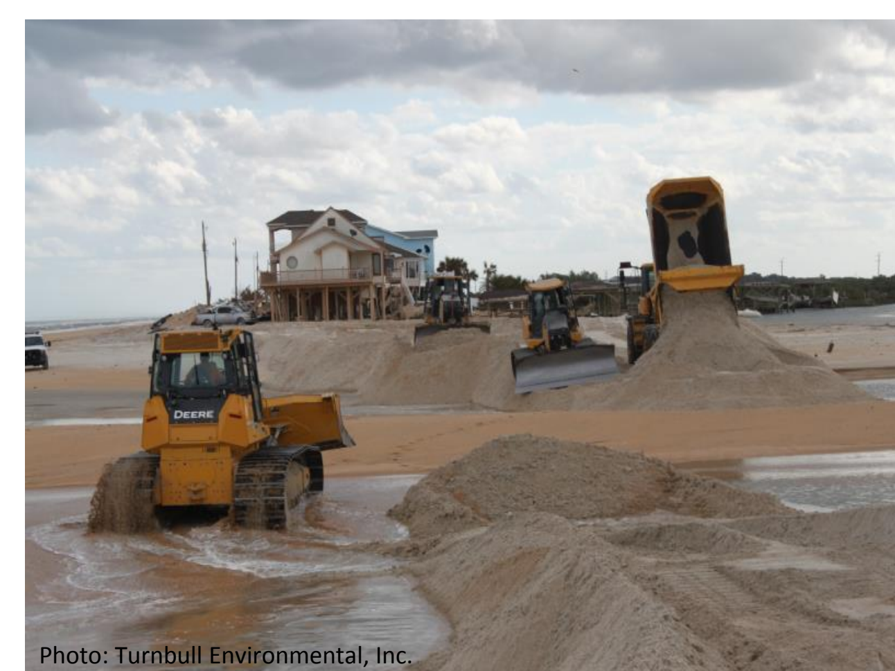
Figure 6 Closing dune breach
