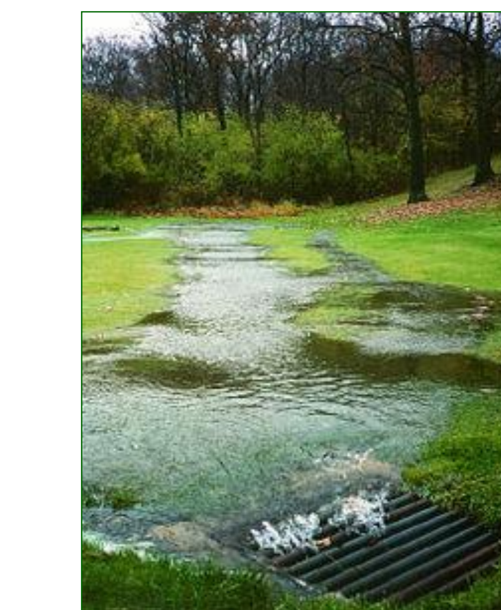
Water runs off saturated soil into a storm drain.
