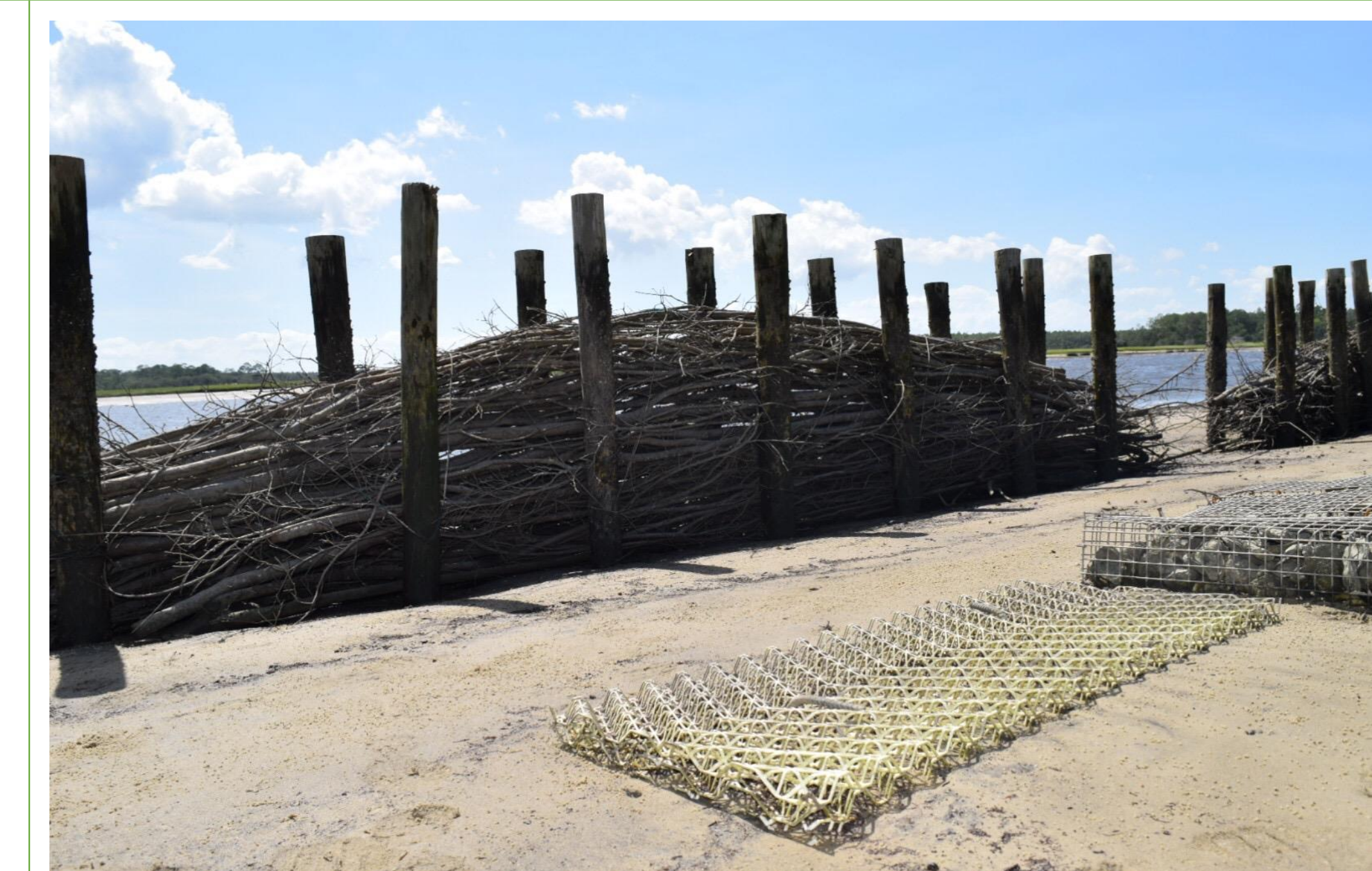
Figure 11. Example of a wooden break wall, a shoreline protection structure constructed with crepe myrtle branches.
